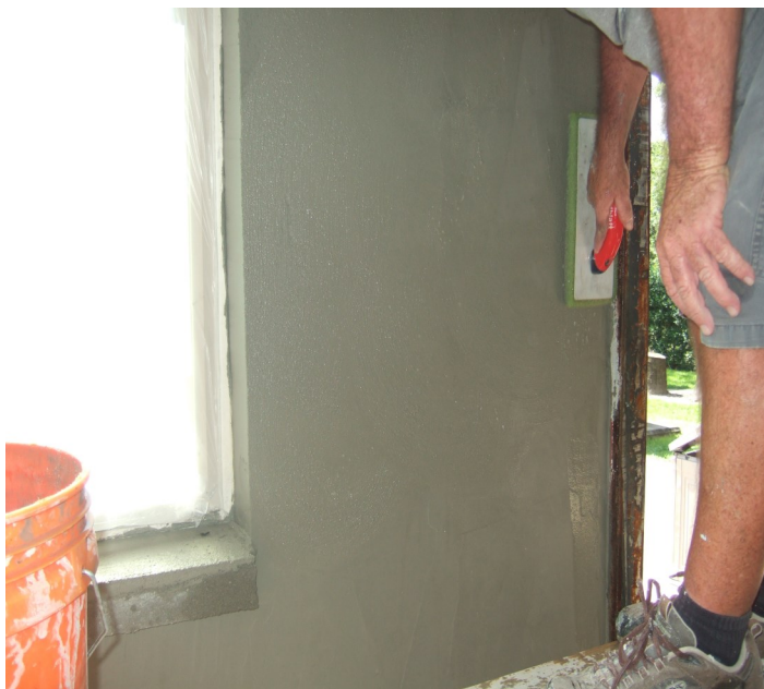
Figure 8-17 Using a soft closed cell float (slide up and down) to gently form a slightly rounded corner.
