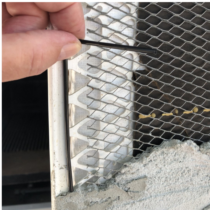
Figure 8-3 - Coffee stirrer shown above slid down into the cavity created by Vinyl Corner Bead's Nosing/Flange Intersection area
