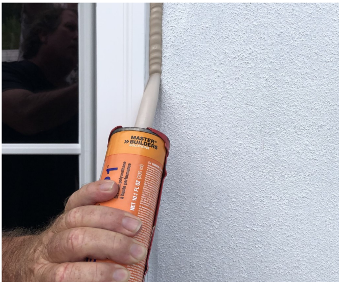
Figure 7-10 Application of Approved Sealant
