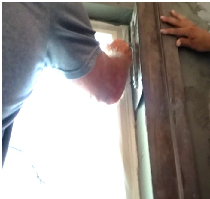
Figure 8-14 Rod set on Jamb Side of the Window Return. Mudding in the return - top to bottom.
