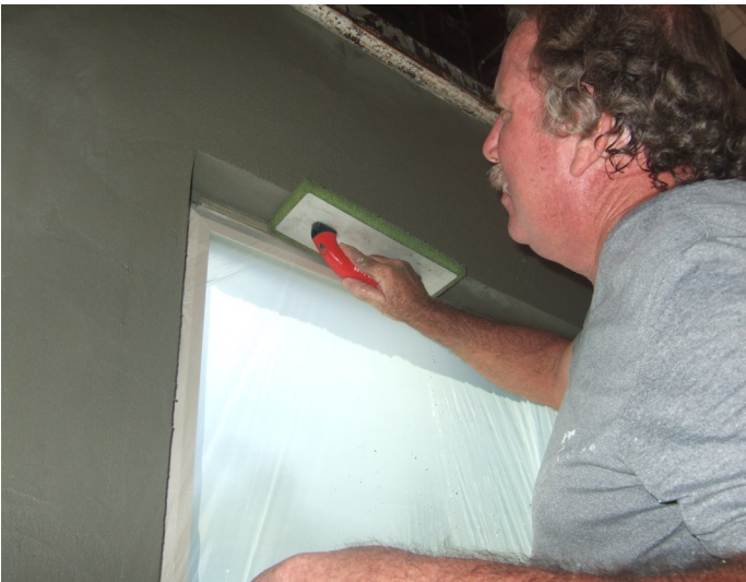
Figure 8-11 Floating the Arris and Window Returns. These are to remain floated and then coated with Drylok. No texture, spray or other impediments to drainage permitted.
