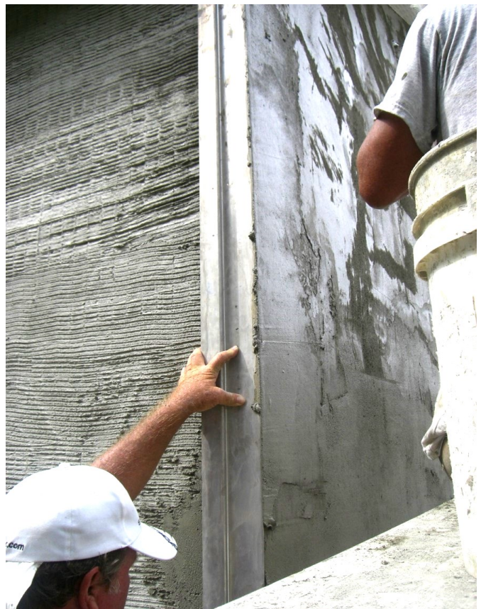
Figure 8-9 Using a Feather Edge Rod to form an External Corner. "Rodding a Corner".
