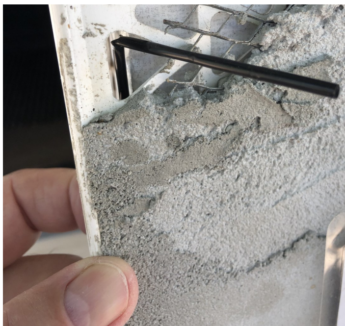
Figure 8-3 - Coffee stirrer shown above slid down into the cavity created by Vinyl Corner Bead's Nosing/Flange Intersection area
