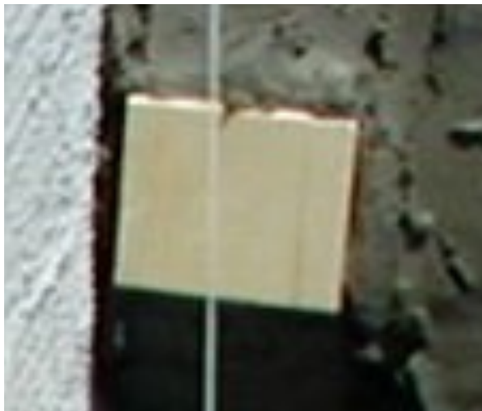
Figure 9-2 Setting "Dots" to a line for Dot-and-Screed straightening. Alternate to control joint screeding.
