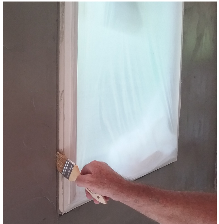
Figure 8-21 Brushing the "V" socket to smooth edges, clean shoulders and seal for application of tooled sealant on frame wall with fin window
