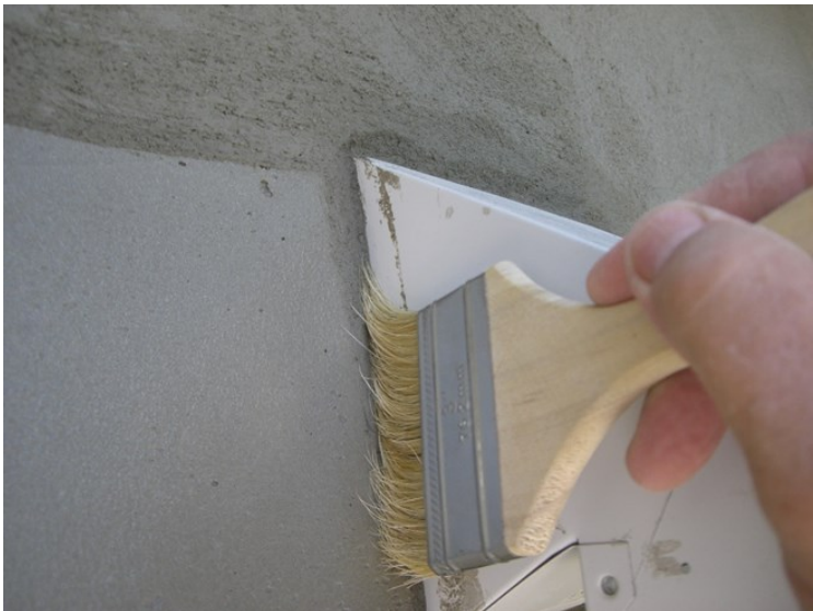
Figure 7-8 After "V" Tooling, the Sealant Socket must be brushed with a brush having dampened bristles. Smooth Edge and Clean Shoulder
