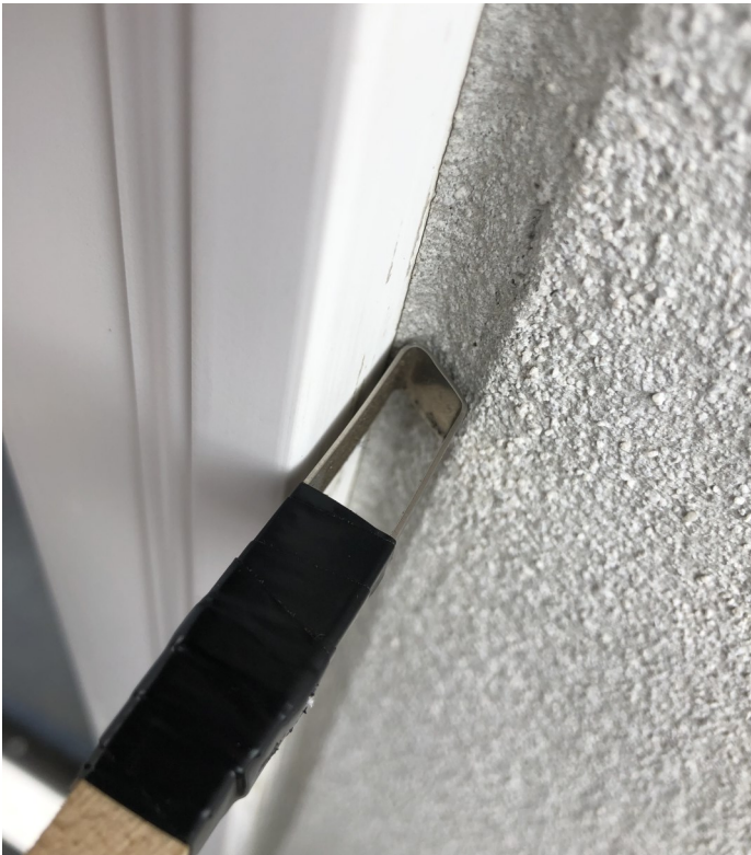
Figure 7-6 Example of Proper "V" Tooling, Brushing, ready for application of Sealant with Spatula
