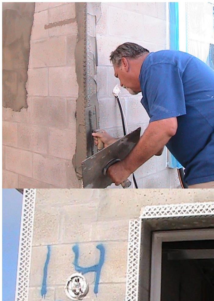
Figure 8-4 - Author demonstrating how to properly "prep" a corner bead to eliminate backside voids. Bead applied to a concrete block wall.
