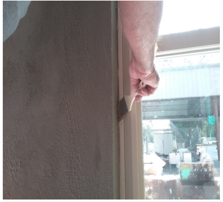
Figure 8-21 Brushing the "V" socket to smooth edges, clean shoulders and seal for application of tooled sealant on frame wall with fin window
