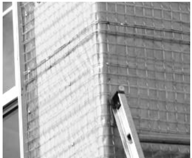
Figure 8-7 StructaLath Wire Bent Around Corner as a Continuous Application
