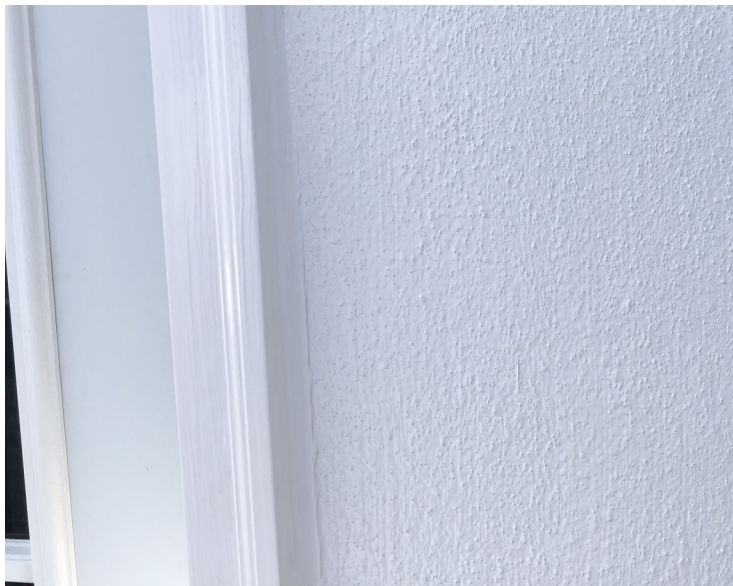
Figure 7-13 Photo of Tooled Sealant Socket after Application of Final Coat of Wall Coating
