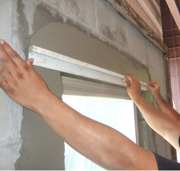
Figure 8-10 Setting a Rod to mud the "arris" (top angle return to the window)
