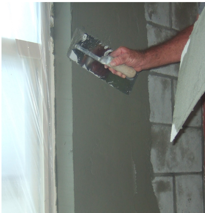
Figure 8-15 Rod "slid off" (upward and outward motion. Trowel removing rod slide-off marks.
