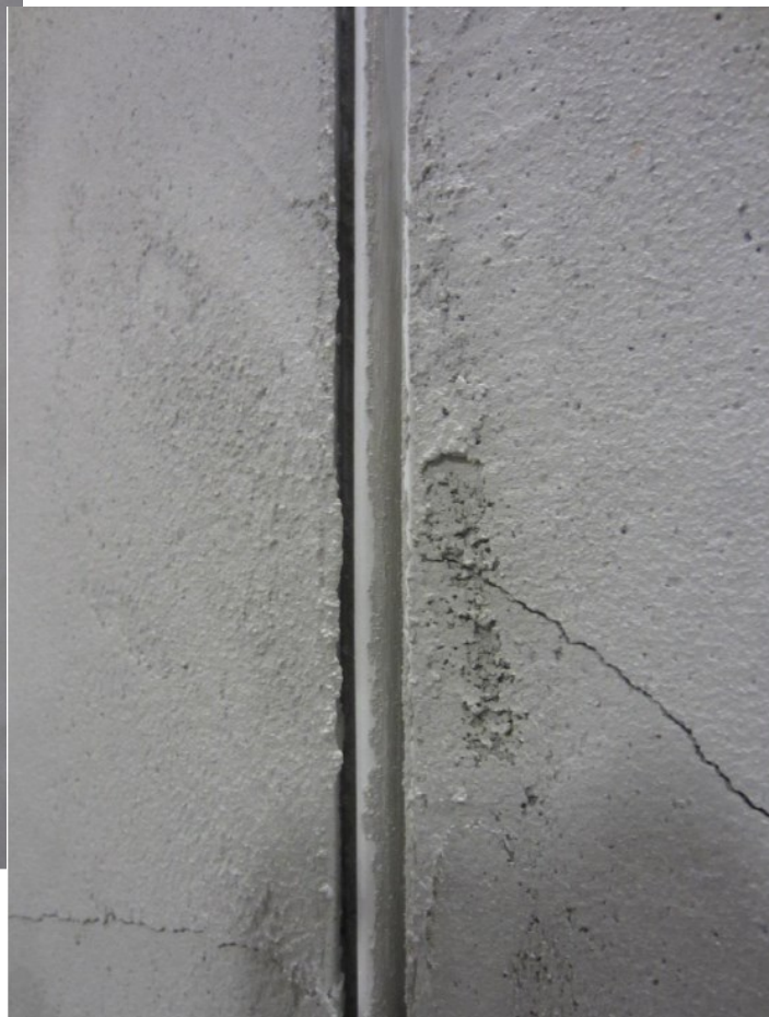
Above - Wall Failure between vertical framing members where fasteners are spaced 16" horizontally - intermediate fasteners needed.
