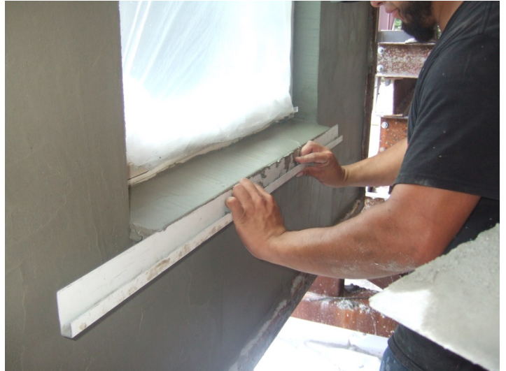
Figure 8-12 Using a Rod to mud the sill to the required slope. (See Detail 06_06)
