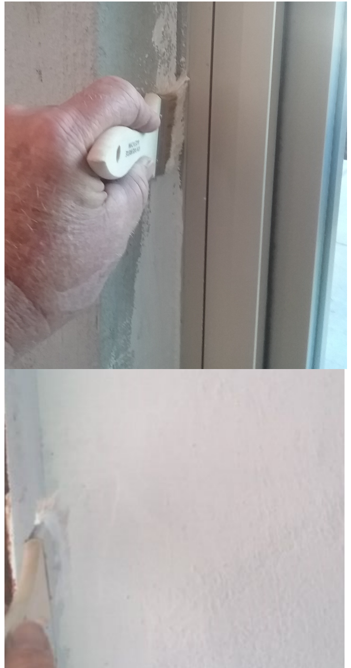
Figure 10-2 Brush Drylok Extreme into all "V" Groove Sealant Socket Seats, Around all Penetrations and along all Shoulders or Stops.
